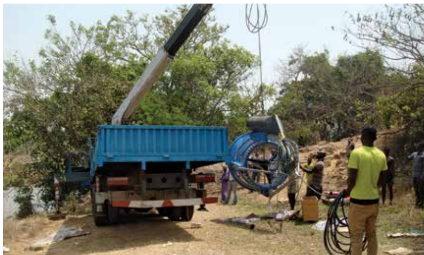
▲ Turbine installation, Nigeria – Credit: Smart Hydro Power
